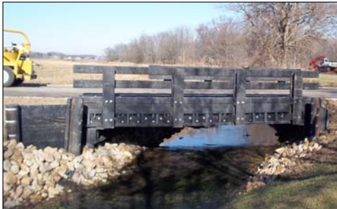
Bridge 174-0.56 over the Onion Ditch
